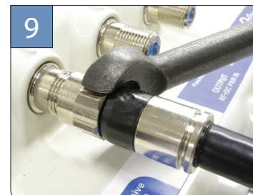
9 Tighten connector to recommended torque.
