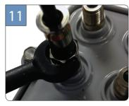
Tighten connector to recommended torque.
