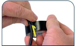
4. Tape the last 4 inches of the strength member onto the cable. Spiral wrap the tape a short distance down the cable, leaving one end of the tape available for removal.
