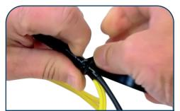
2. Secure mesh edge with tape, catching a small amount of the cable (approximately 1 inch).
